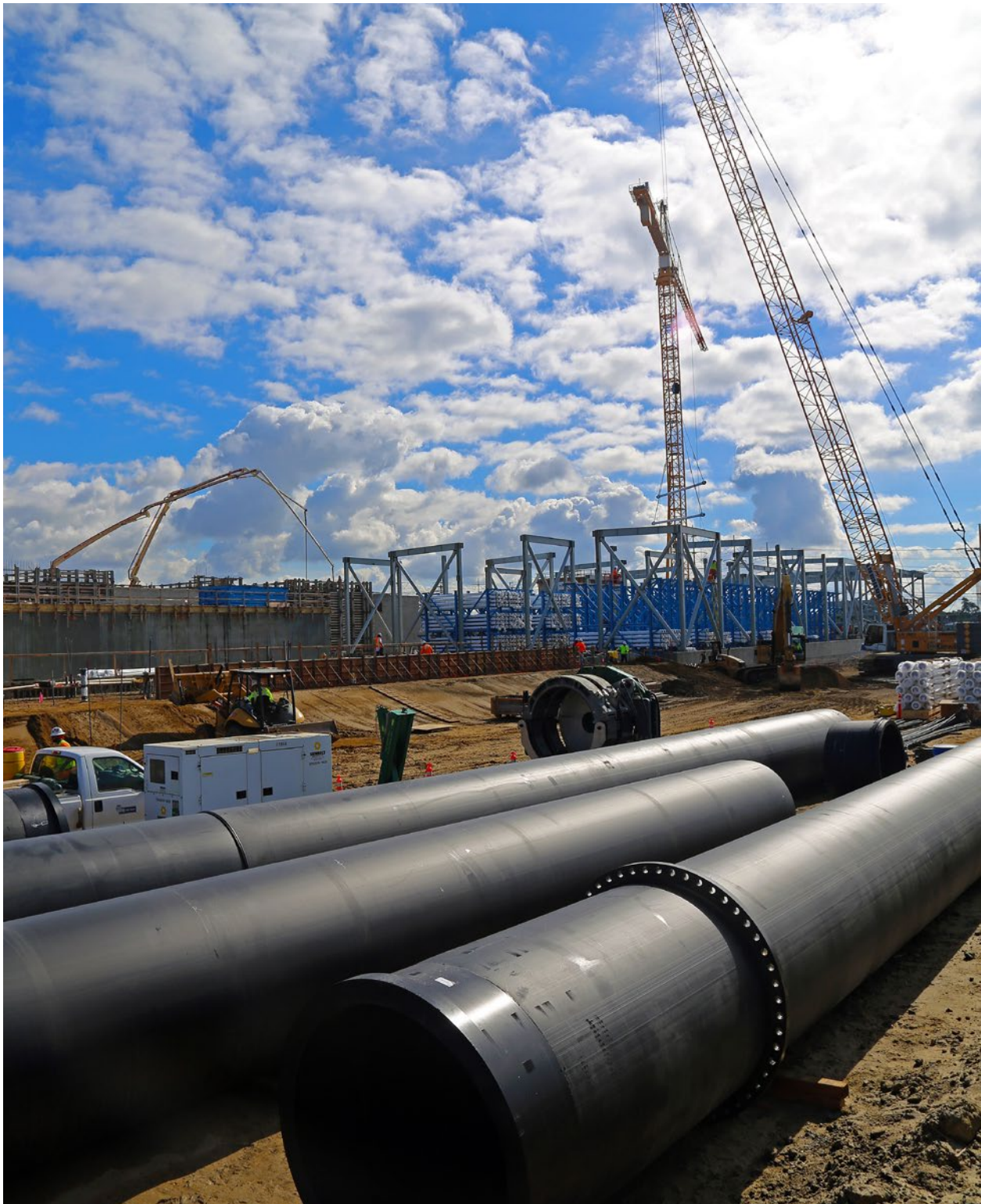
San Diego County Desalination Plant: www.isco-pipe.com/SanDiegoCounty
